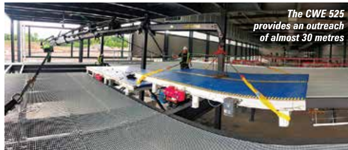
County Lifting's CWE 525's was recently used to assist with the installation of flooring
