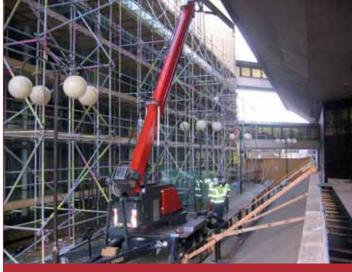
GGR was able to provide the Royal Bank of Scotland with a Skyworker crane after several other crane companies had to turn the job down. The Skyworker overcame restricted access problems and the need to reach over the top of the building to install the canopy glass.
