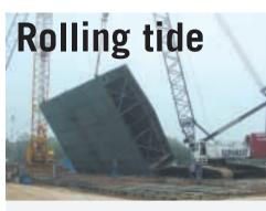
MASTER BOAT Builders Inc of Coden, Alabama, US, relied on the powers of Barnhart Crane & Rigging to roll three massive components to be used in the construction of a crew boat set for duty in the offshore industry. Barnhart called on two of its Demag crawler cranes for the job, a 544 tonne capacity CC2600 and a 299 tonne capacity CC2000, to "bookend" each of the three sections of the boat, the heaviest of which weighed 290 tonnes. A fourth component weighing 118 tonnes was then set in place.
