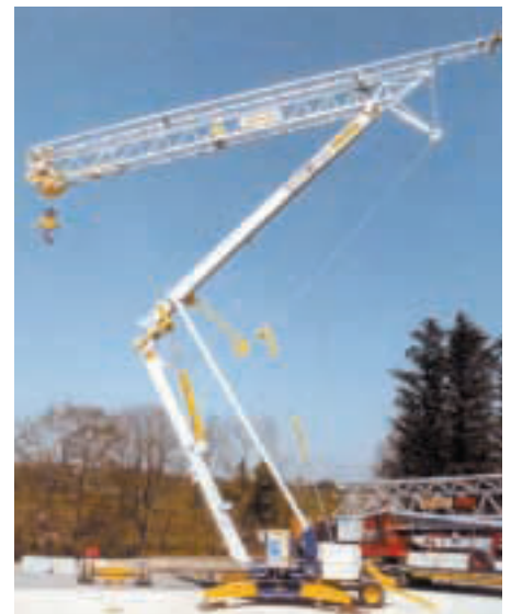
According to Mantis Cranes' Rober Rowlette, "One of the principal benefits of a self-erecting tower crane against a top slewing crane is in costs in terms of both set up and removal, as well as operating costs.
