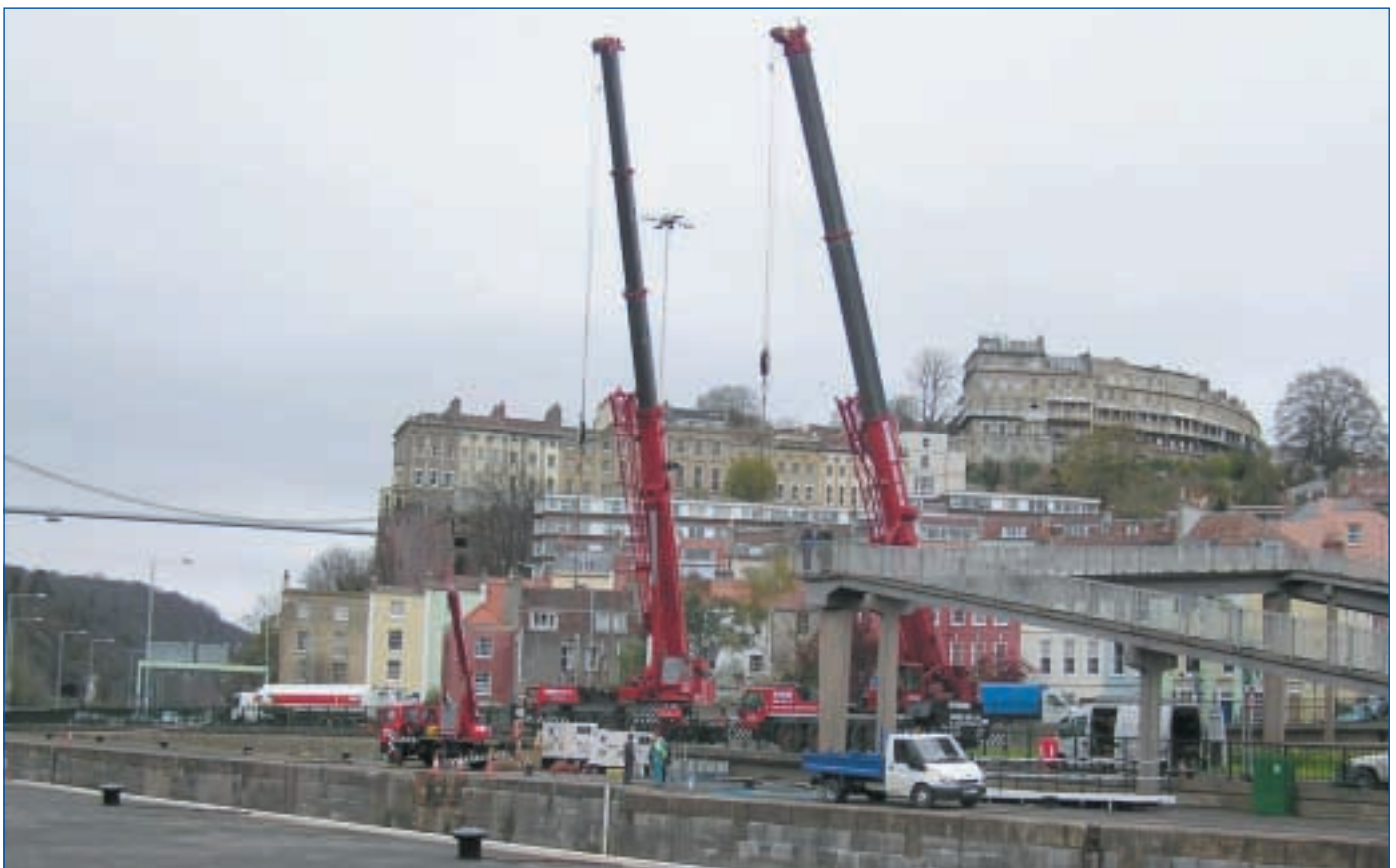
The Clifton Suspension Bridge in Bristol formed the backdrop to a lift performed by Sparrow Crane Hire recently, which was called in by Bristol City Docks to assist in the re-fitting of 90 tonne lock gates at the Cumberland Basin in the Avon Gorge. For the main part of the lift, Sparrow brought in a 100 tonne capacity Grove GMK 5100 and an 80 tonne Liebherr LTM 1080/1, (pictured), while supporting roles were provided by two Demag AC 40/1s and a Tadano TL 75.
