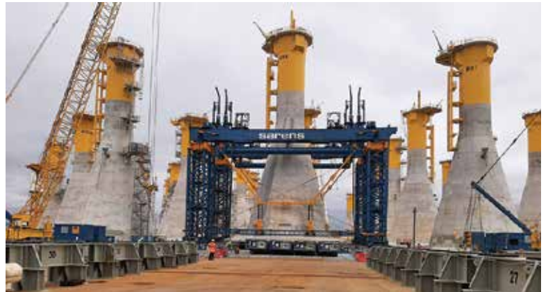
Each of the 71 concrete structures has a 31m diameter base, is 48-50m high and weighs 4,800 tonnes
