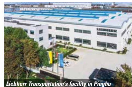
Liebherr Transportation's facility in Pinghu
