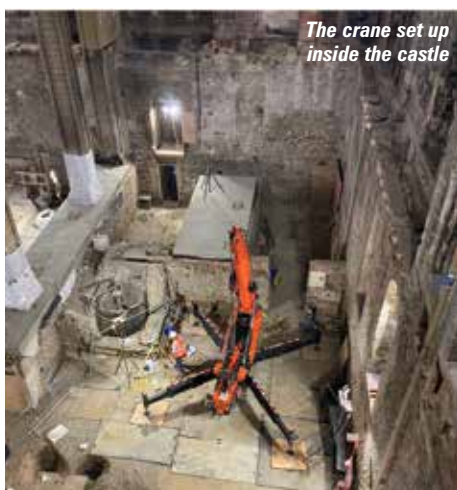
Asa Wilkinson uses the remote on his Jekko SPX 650 at Norwich Castle
