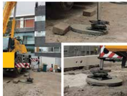
Some of the examples found on site
