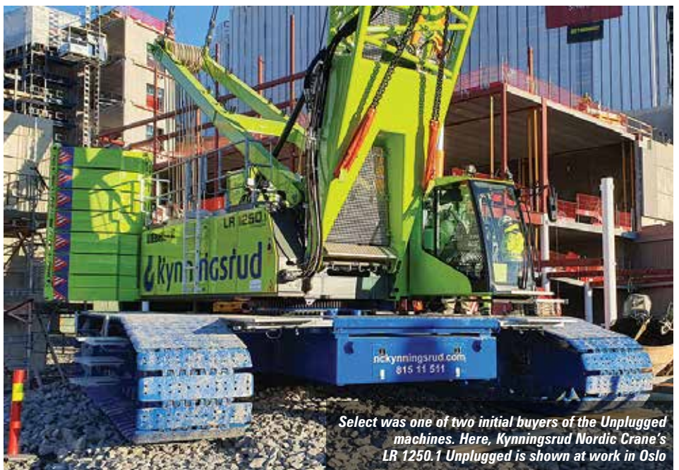
Plugging in the Liebherr Unplugged crawlers at Old Oak Common
