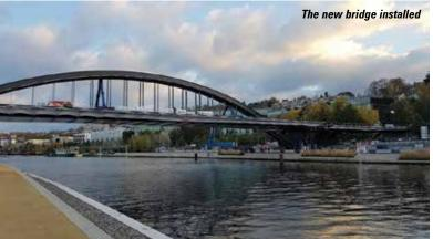
bridge from the quay to the barge and span the 15 metre gap, while extending the effective barge width. The assembled bridge spans were then able to be transferred aboard. This required the carefully choreographed use of 84 axle lines of SPMTs along with the jacking towers, to manoeuvre the spans onto the barge, float them out and then position them. The new bridge is due to open to traffic this summer. *See the video https://www.youtube.com/ watch?v=tU7ysT7lXyc*
