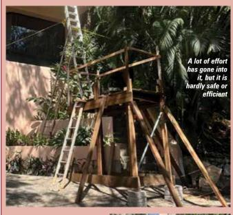
Spotted in Acapulco, Mexico, men painting a series of buildings with equipment and methods that make the job harder, slower and less safe. Most work was at a height of nine metres or so and the hard standing below is sloping. Rather than using a tower, or trailer lift etc the contractor has constructed wooden staging levelled with bricks and topped by long ladders. A lot of effort has gone into it, but it is far from safe or efficient.
