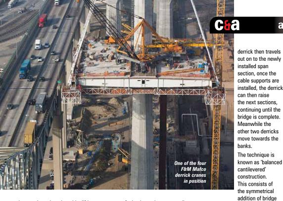
it extends to the other side, lifting materials and span sections from barges below or from road transport.
