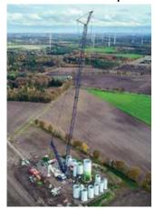
SL10DF2BV wind power boom system. The 168 metre main boom and fixed offset jib of up to 24 metres provides
