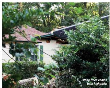
Similarly, on a normal lift a competent operator will add the load to the hook gradually. Taking a tree section at height applies the full load instantly, possibly with an added dynamic loading, which can both take the lifting device over its safe working load and introduce stresses across the equipment for which it may not have been designed. Slewing gear and telescopic booms are also not built for the regular side loadings or bounce that can occur in tree work.
