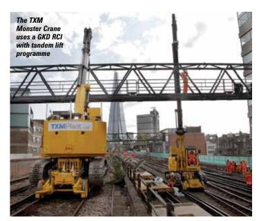
overpass. The 'Monster Crane' lifted each structure from a tractor trailer at a safe location and then caried the load along the line with a one in twenty gradient, while trains continued to travel at full speed on the adjacent line. This enabled the job to be completed in 12 weeks. The traditional solution would have involved a 400 tonne crane lifting the loads across the tracks, requiring it to be shut to trains. The severe limits on the time available for closing lines would
