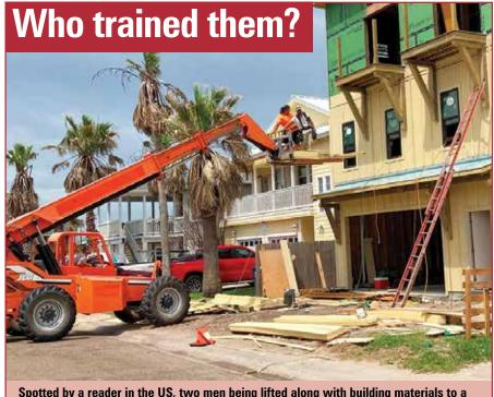
Spotted by a reader in the US, two men being lifted along with building materials to a second storey balcony on the forks of a telehandler. Also note the state of the site and that ladder!
