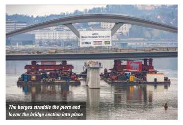
2,800 tonne bridge segments from their pre-assembly height to the load out height and then float them out to the adjacent piers.
