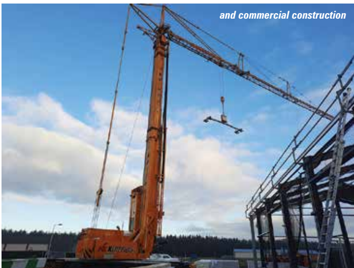
Cranes are used intermittently at key stages in housebuildings...
