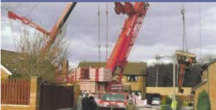
Crane Services to the rescue with 900 tonnes of lifting capacity.
