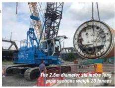
boom angle. The crane offers a capacity of 55 tonnes at six metres radius, or 20 tonnes at 12 metres.
