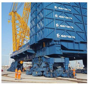
SGC-250 the crane was rigged with 118 metres of main boom and 52.3 metre luffing jib ready for its first major lift. Fitted with a custombuilt 700 tonne Sparspin spreader system, which allowed for six pieces to be individually controlled during a lift, the crane worked through the night to lift the 170 tonne prefabricated dome on the reactor's steel containment liner.
