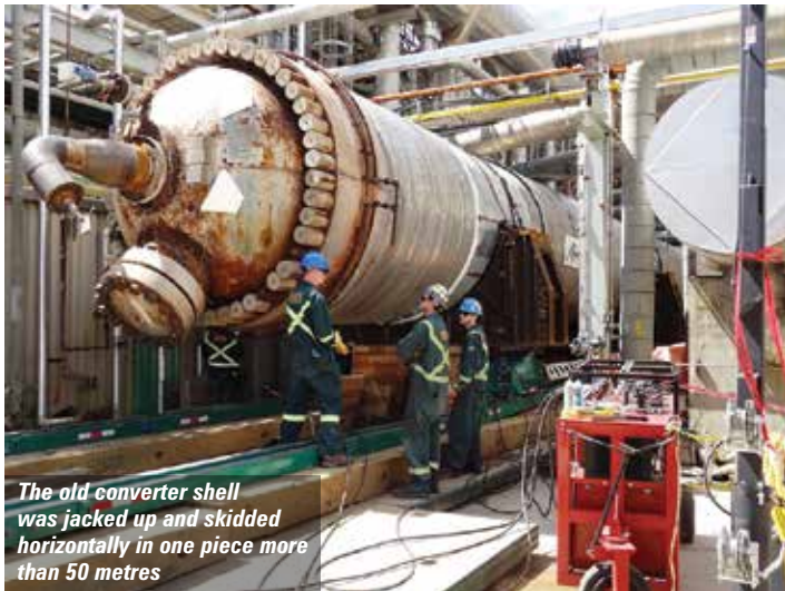
The Hydra-Pac synchronous hydraulic unit powered six JSL250 jacking load shoes, allowing even weight distribution and load compensation, even with poor ground conditions
