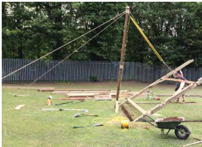
The Gin Pole is rarely used these days but still has its place.
