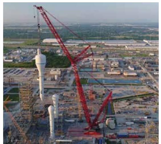
Mammoet used just one heavy lift crane - a 3,200 tonne Liebherr LR13000 - at Braskem's new $675 million Gulf Coast polypropylene plant at its Delta facility in La Porte, Texas.
