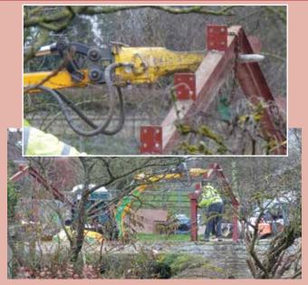
Spotted in the UK a demolition contractor dismantling a steel frame building using an excavator and breaker for all the lifting. As they removed the bolts from the joined roof truss, it rotated on the breaker tool wildly, almost knocking one of the men in the head and brushing the other off the wall he was standing on.
