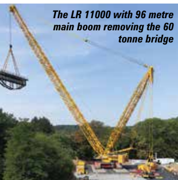
Two arched fish-bellied girders under the bridge support, had to be removed before being placed on the ground
