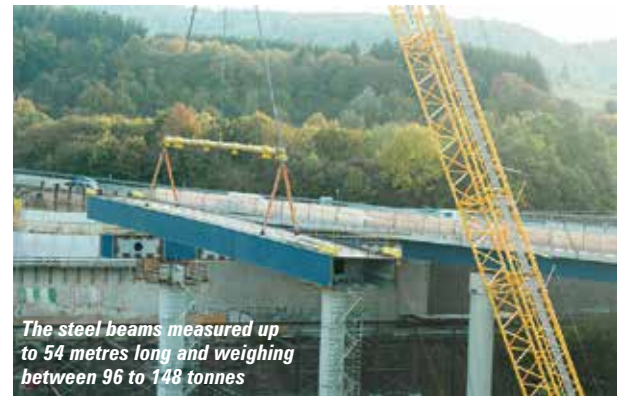
Wiesbauer used its Demag CC 3800-1 to replace the old viaduct on the A45 highway that spans the river Lahn near Dorlar, Germany
