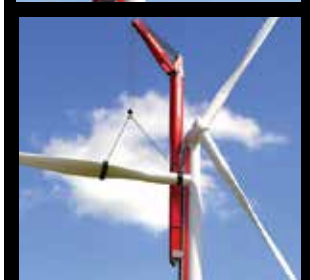
The Mammoet WTA 250 attaches to the base tower and installs the rest as it climbs its pre-installed track
