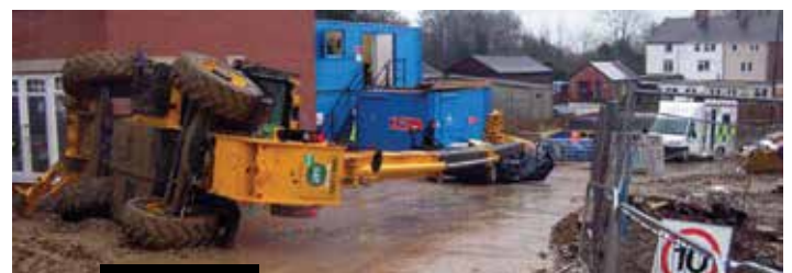
Carrying a suspended load is particularly dangerous for a telehandler
