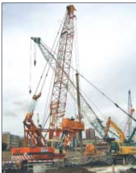
An IHI DCH800 working with a Soilmec RT3/ST rotary drilling rig
