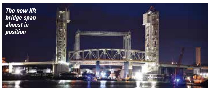
The bridge span was floated into position
