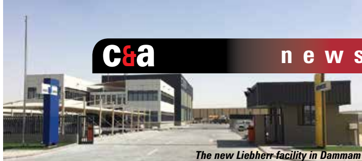
The new Liebherr facility in Dammam
