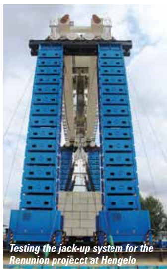
Transporting the 2,400 tonne capacity gantry crane
