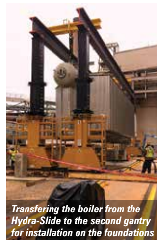
Once the boiler was off the railcar it was lifted by a Grove GMK 7550, slewed through 90 degrees and installed on the skidding system
