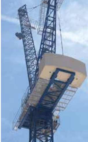
Comansa CM's first luffing jib tower crane
