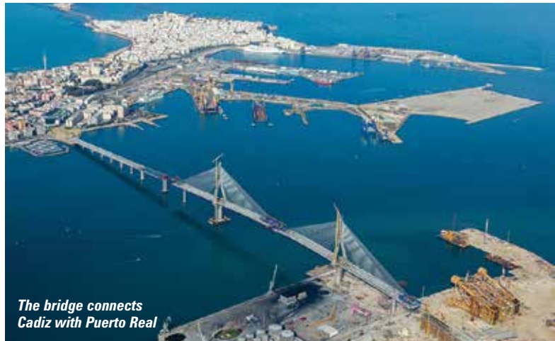
Total length of 'La Pepa' is 3,092 metres and is one of Spain's largest infrastructure projects in recent years
