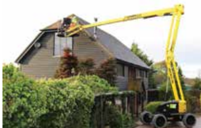
Facelift has taken delivery of 30 Niftylift HR17 boom lifts
