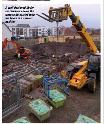
lifting and travelling with suspended loads is generally more hazardous than lifting unit loads on the telehandler's forks.
