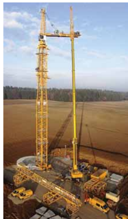
One of the main advantages of using a tower crane is the reduced amount of space needed to erect the crane.
