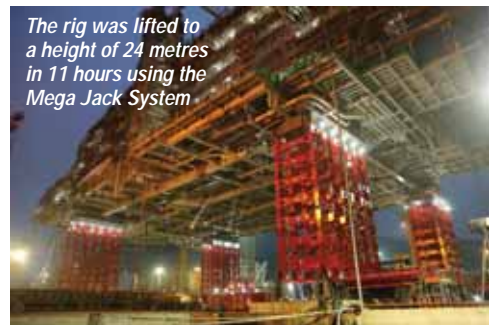
The load comprised the topside for a new ice-resistant fixed platform for an offshore platform
