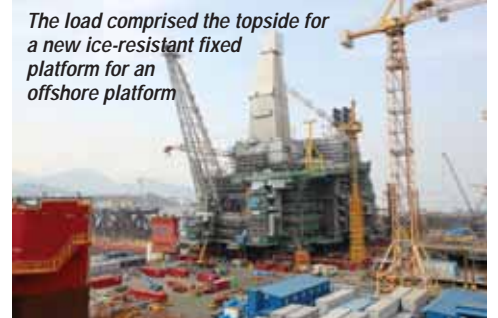
Each corner - made up of three towers - had a capacity of 15,000 tonnes
