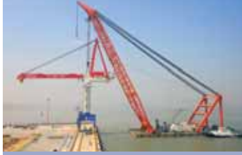
Huisman China installs a 2,400 tonne quayside crane at its fabrication yard in Zhangzhou.
