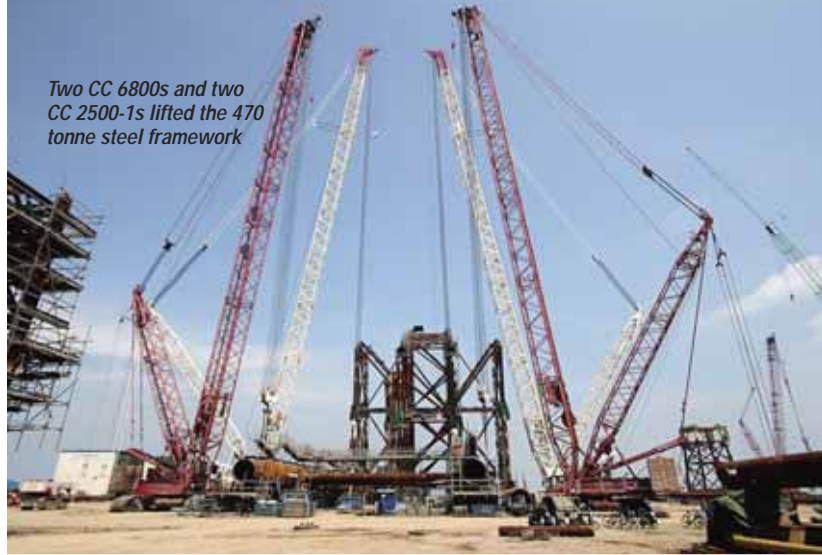
The frame was carried 75m into position...
