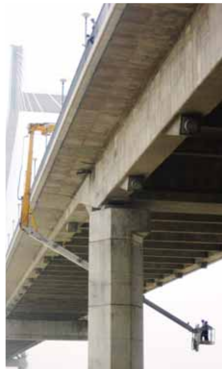
A podium type tower or electric/pneumatic powered telescopic AWP type platform can give additional work height above the platform
