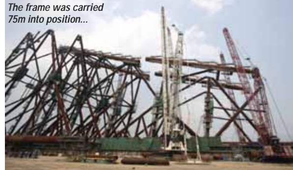
...before the sections were brought together
