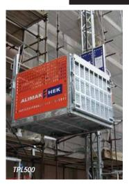
offer dual functionality for use as either a transport platform or material hoist and conform to the latest safety standards featuring an overload protection and over speed safety device.
