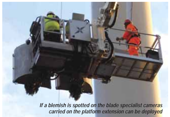
A dirty blade is cleaned and inspected all in one sweep
