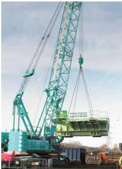
A Kobelco CKE1350G on site in Beckton, East London rigged with 30m of main boom, lifting 55 tonnes.
