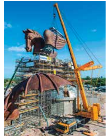
A seven axle, 400 tonne Liebherr LTM 1400-7.1 AT crane operated by Allegiance Crane of Pompano Beach was used.
