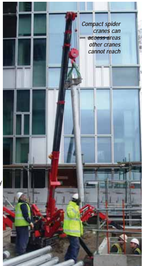
Two spider cranes solve a lifting problem at Addenbrookes Hospital, Cambridge
