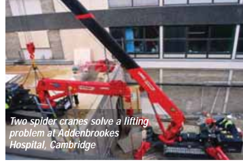
Compact spider cranes can access areas other cranes cannot reach
