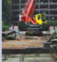
Heavy duty crane access mats
