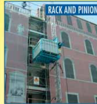
MAST WORKING PLATFORMS
