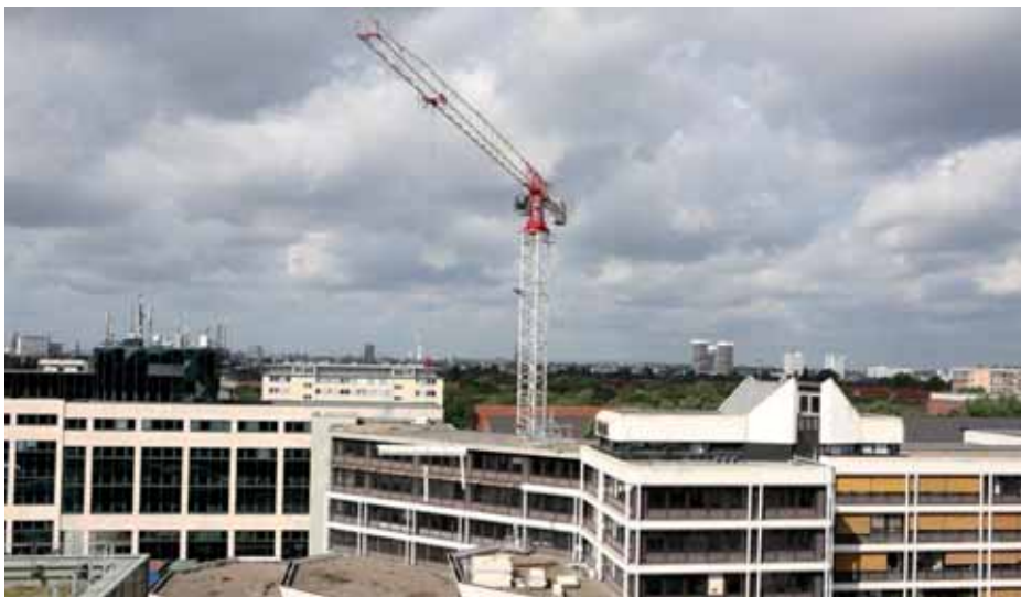
The first climb of a Jost crane.
