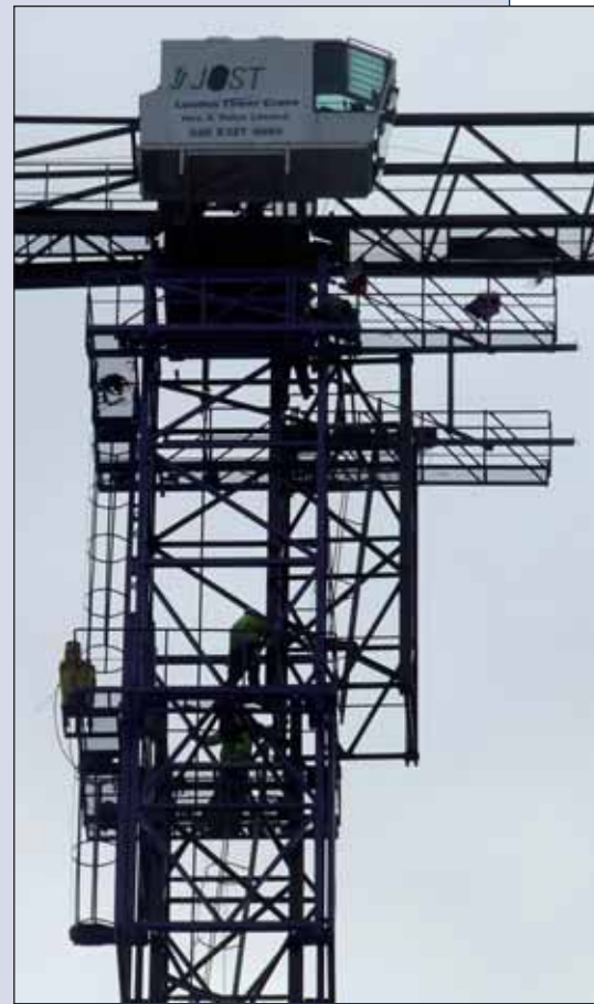
The first climb of a Jost crane.
