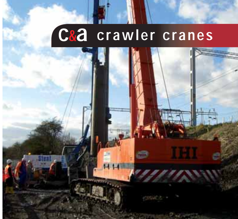
An IHI CCH500T working as a service crane lifting casings for a Stent piling rig working alongside the railway in Rugby. The unit was specified in order to mitigate the risk of the boom falling over the live line and has a slew restrictor fitted in order to stop the operator from inadvertently slewing over the railway.
