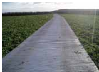
Eve Trakways new K panels form a temporary road over farm land.
