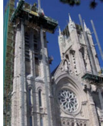
With Mastclimbers tourist attractions/city landmarks need not be covered in scaffold for years.
