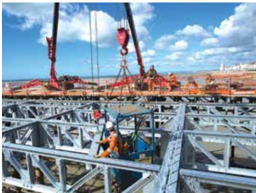
Unic 706 spider cranes from Coppard Plant have been helping replace 500 deck beams and 350 lattice girder beams.
