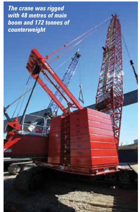
The first Manitowoc MLC300 working on a Wisconsin highway project
