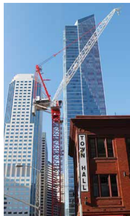
The 700B will climb externally to 233 metres using 23 tower sections and 10 tie-in points - compact dimensions and quiet operation make it ideal for the downtown site.
