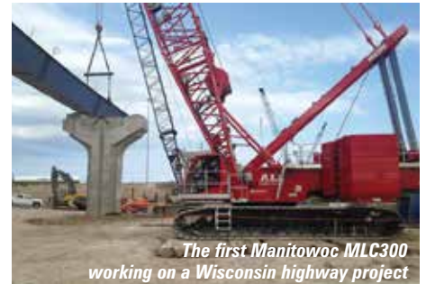
The crane was rigged with 48 metres of main boom and 172 tonnes of counterweight
